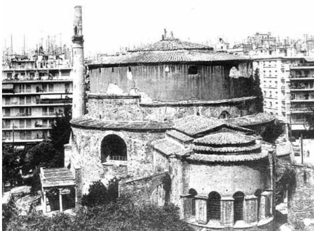
Fig. 1. Rotunda, exterior view (photo: N.K. Moutsopoulos).
