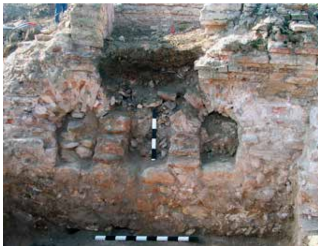
Fig. 6. Detailed picture of the suspensura in room Nr. 1 of late antique bath;
