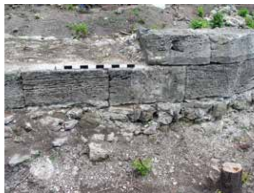
Fig. 14 Quadra blocks from the plinth rows of Tower No 8, the western fortification system of Bononia .
