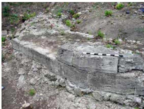
Fig. 12 Construction of the walls of Tower No 8 – quadra and brick rows.
