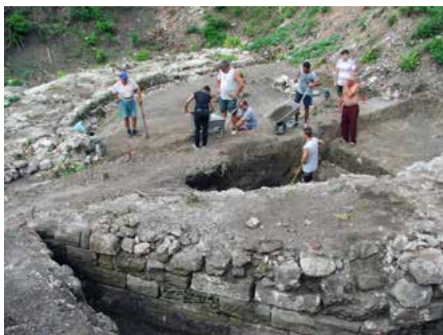
Fig. 8 The beginning of the excavations of Bononia 2014 – inside Tower No 8.
