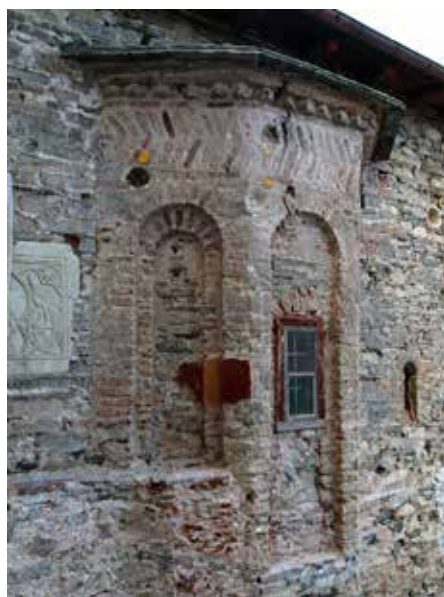
Fig. 3 Chapel of Hagioi Anargyroi, monastery of Vatopedi, Mount Athos. Eastern wall and apse after the removal of the plaster (photograph: P. Theocharides)
