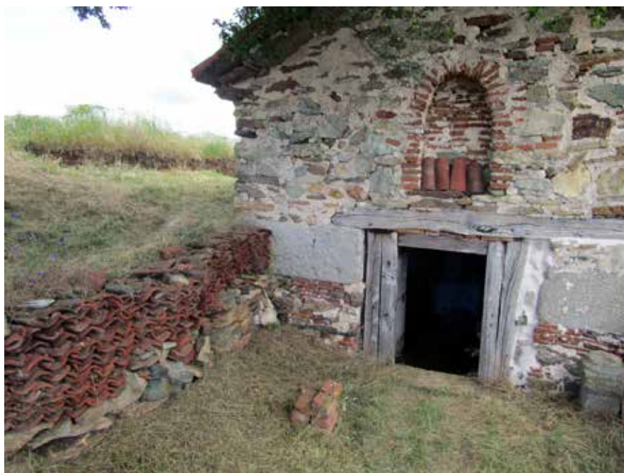
Fig. 15. The western wall of the church. Built, with reused bricks and tegulae .
