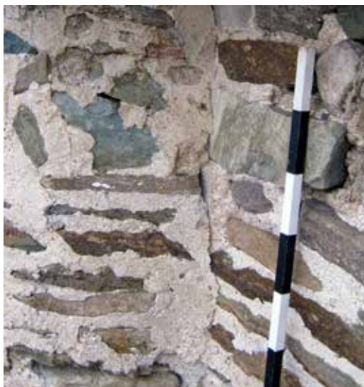
Fig. 16. A gap between plastered south wall and the later built conch. Details.
