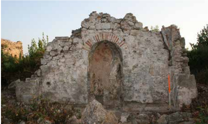
fig. 20 Fountain house, northern front wall © ÖAW/IKAnt (M. Hernandez-Cordero)
