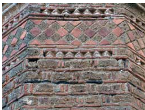
Fig 6. Opus reticulatum, detail from the apse of St. John Kaneo church, photo: Jasmina S. Ćirić
