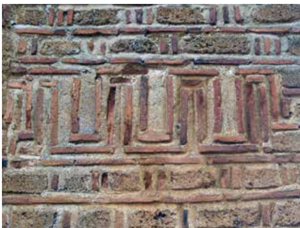
Fig. 10. П meander, details of the apse, St. John Kaneo church, photo: Jasmina S. Ćirić
