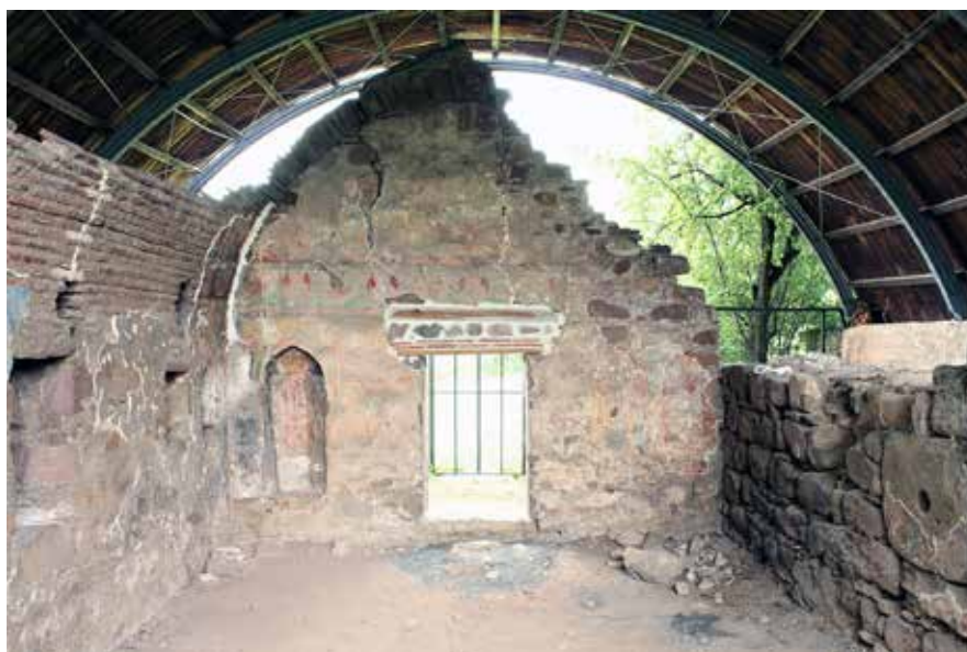
Fig. 8. Western interior wall, 2017.
