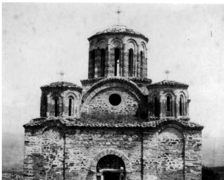
Fig.3. Condition of the Church of the Holy Mother of God, year 1930, photo: Đurđe Bošković
