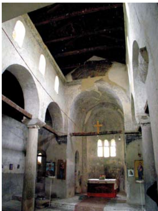
Fig. 2. View to the eastern part of the church.
